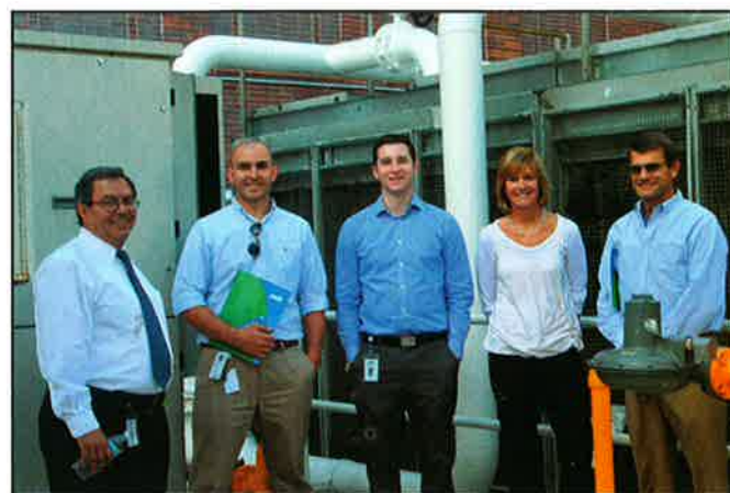
Pictured in front of the Capstone Microturbine from left to right: Sherif Youssef (PGW) , Brad Fitzpatrick (SunGard), Bryan Dallas (PGW), Cindy Overby (PGW) and Greg Konrad (SunGard).
